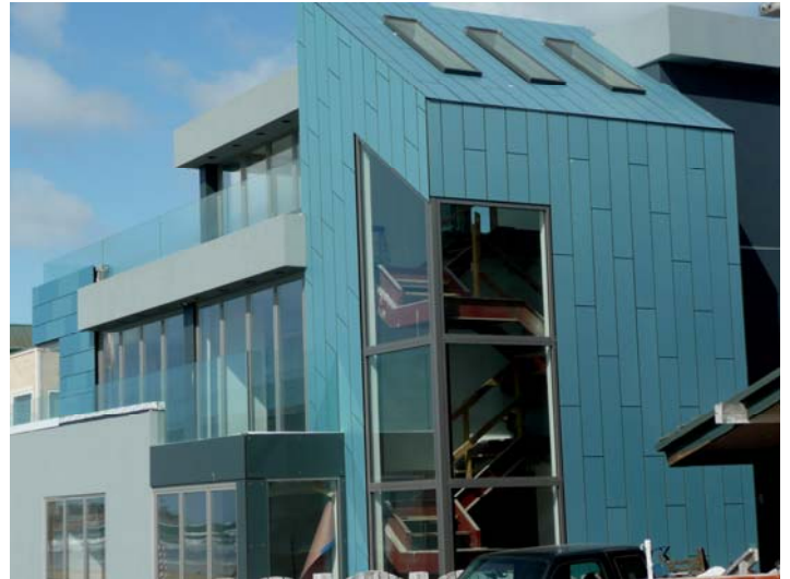
Residence from the Southwest View. This is the ocean front side of the home. WallShield was chosen for the building envelope for its extreme weather resistant properties and ability to prevent mold and mildew.
